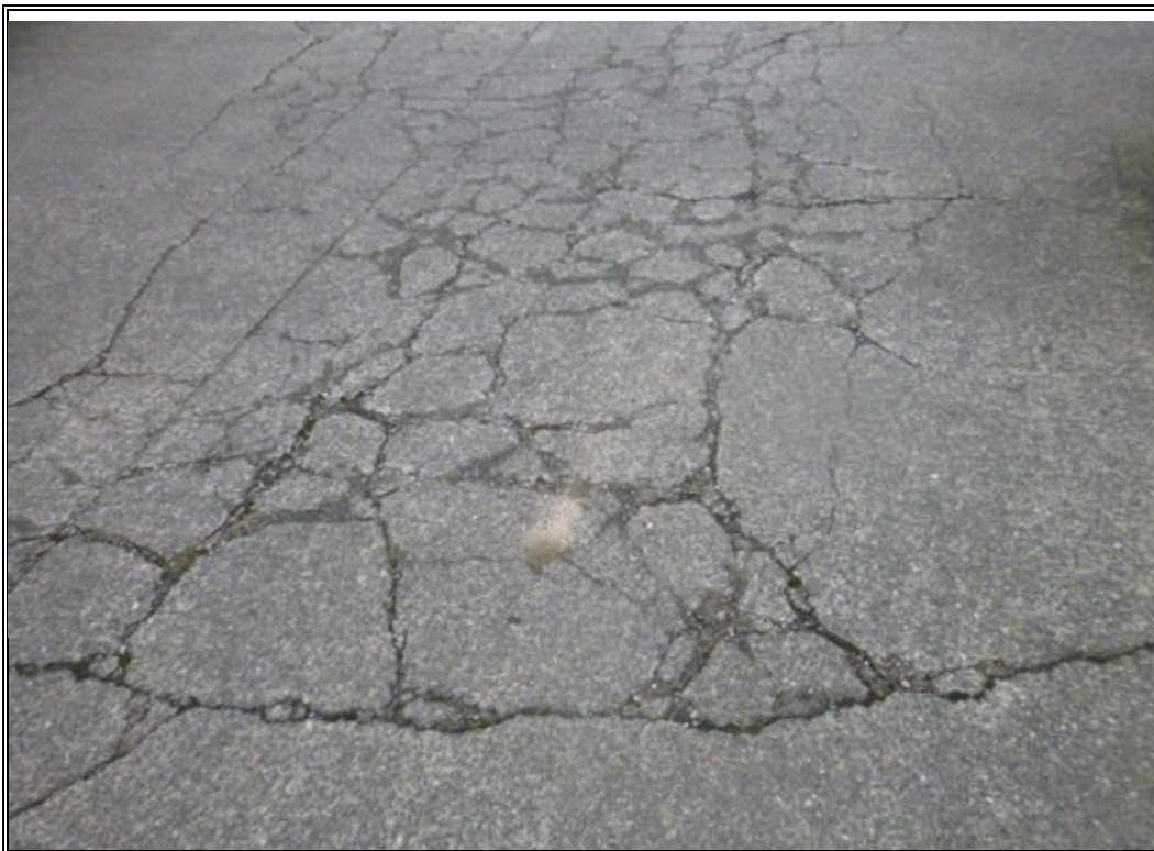
Description: Cracking and distress in concrete driveway access
